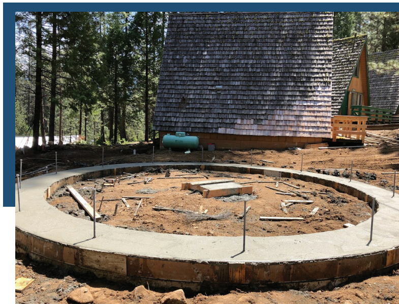
Base for new water tank
