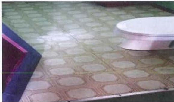
Material: 12" VFT and Mastic - Tan Squares HMR #: 4 Asb: Comment:
