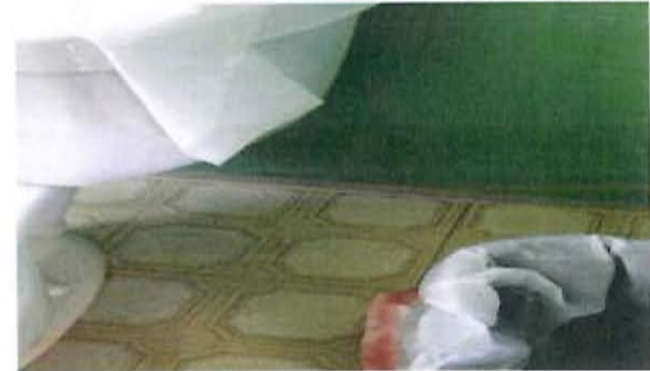
Material: 9" VFT and Mastic - Tan HMR #: 23 Asb: Comment:
