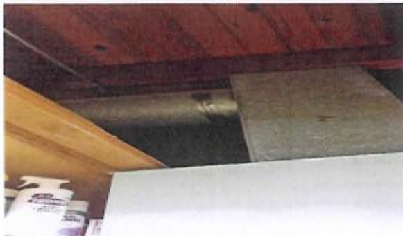
Material: Transite Flue Pipe HMR #: 28 Asb: Comment:
